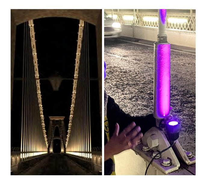
Luminaire with optical control to illuminate the hangers and light the underside of the chains.
