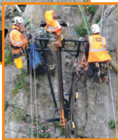
Works on the Clifton Suspension Bridge include rock bolting and (opposite) parapet stanchion replacement
